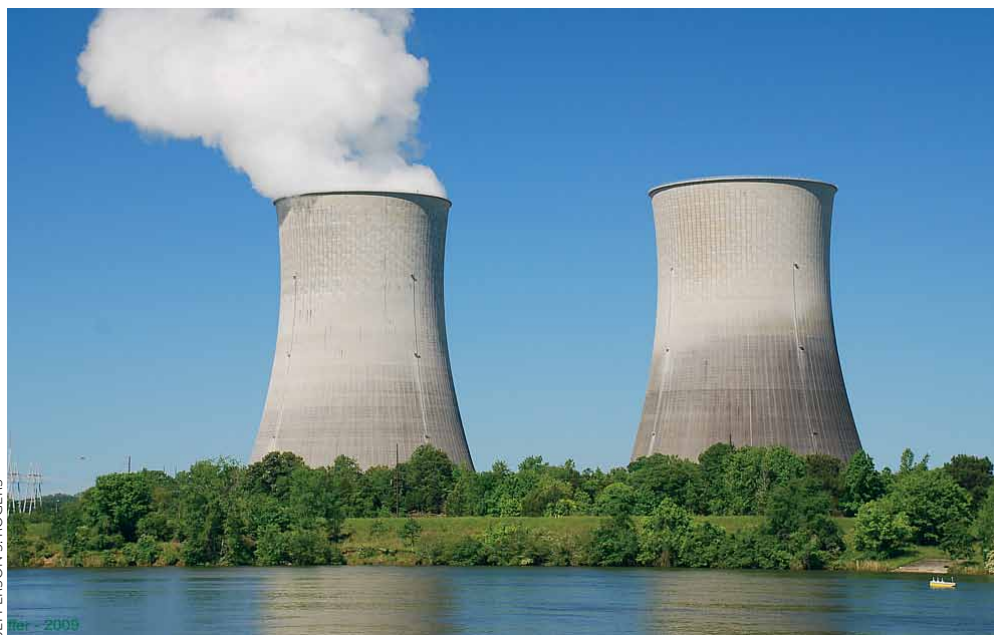
The hot steam generated during nuclear fission is cooled using cooling towers.
